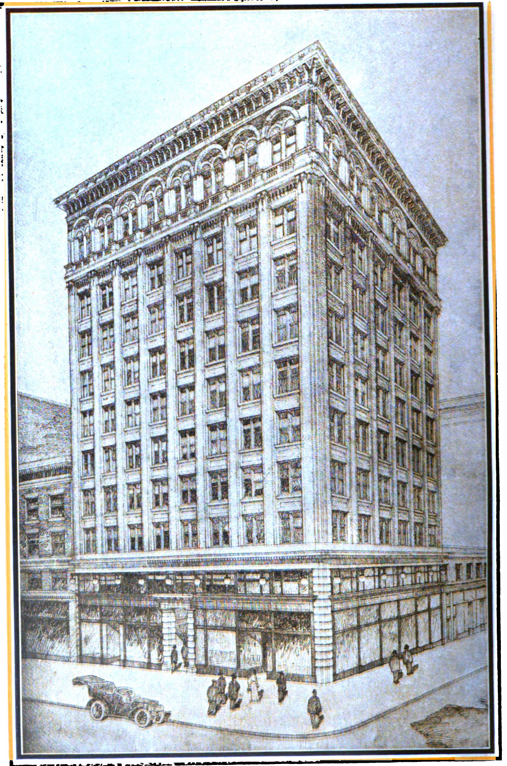
BALBOA BUILDING, A STEEL FRAME OFFICE STRUCTURE, AT MARKET AND SECOND STREETS; OWNER, A. A. MOORE; COST, $300,000; ARCHITECTS, BLISS AND FAVILLE
